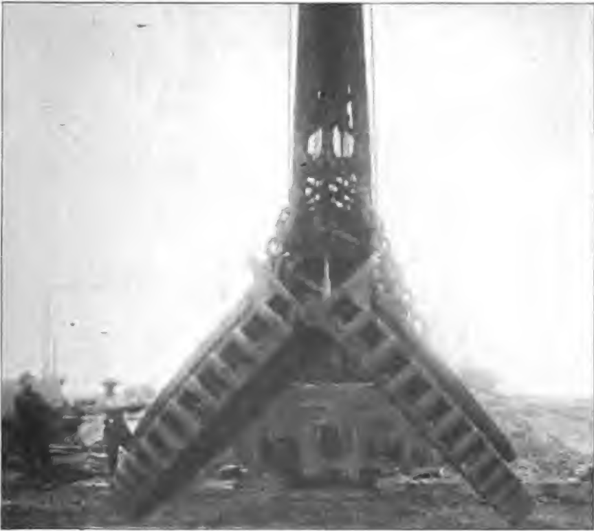
BASE RING OF THE 14-INCH, 45-CALIBER AMERICAN GUN MOUNT, MODEL "E" (THIRD STEP OF INSTALLATION).
